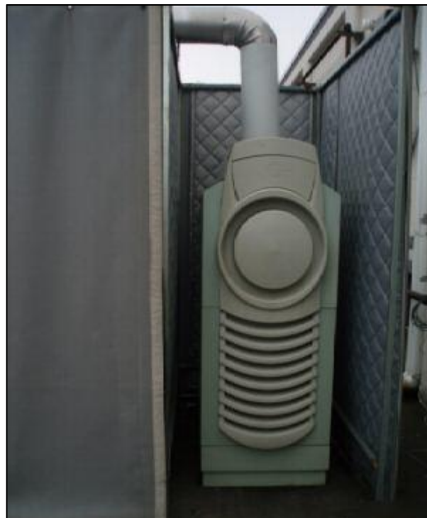
Figure 9: A micro turbine with waste thermal power unit attached
