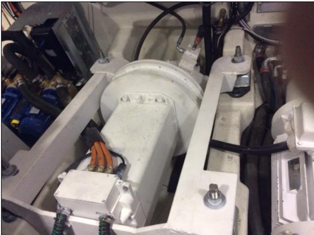
Figure 6: Electric motor on FV Karoline
